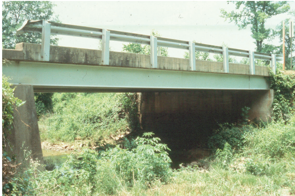
Figure 8.2.1 Simple Span Rolled Multi-beam Bridge
