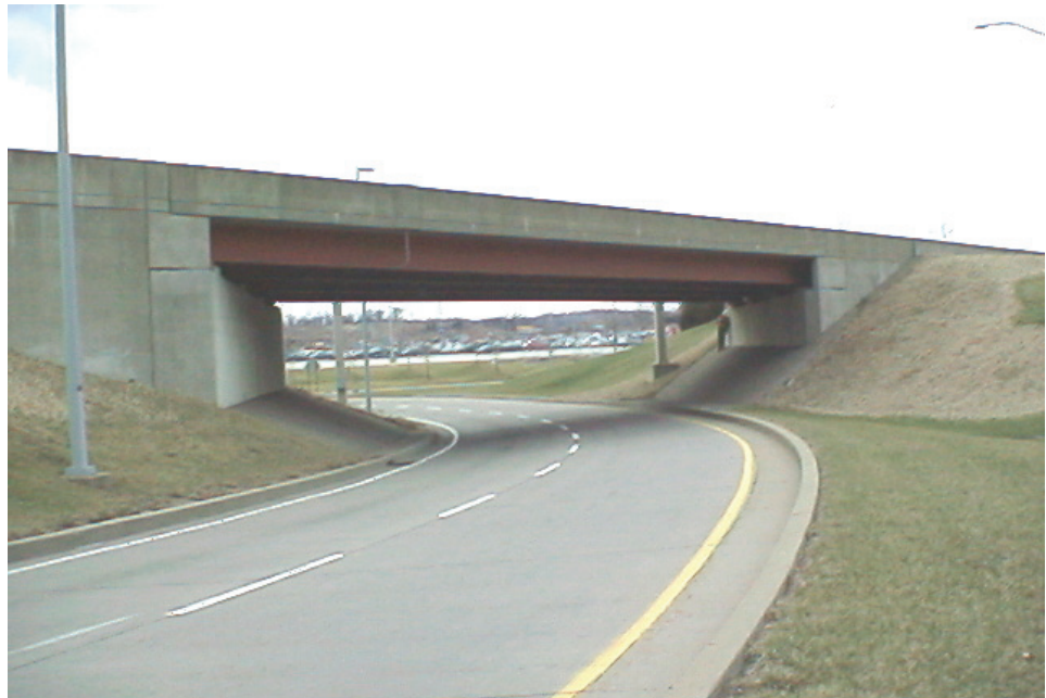
Figure 8.2.6 Single Span Fabricated Multi-girder Bridge
