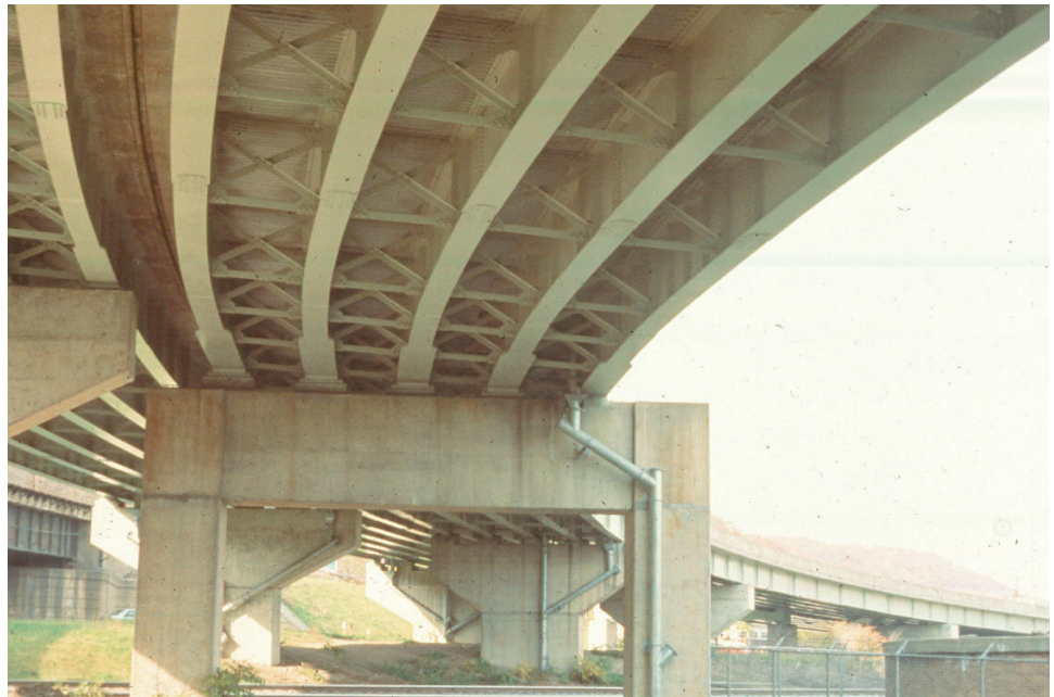
Figure 8.2.8 Curved Fabricated Multi-girder Bridge
