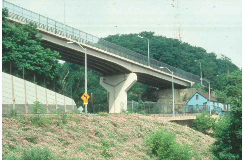
Figure 8.2.7 Continuous Span Fabricated Multi-girder Bridge
