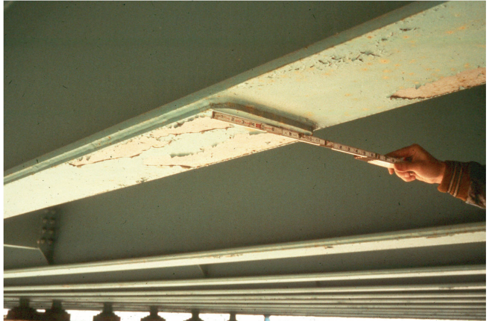
Figure 8.2.3 Rolled Multi-beam Bridge with a Cover Plate
