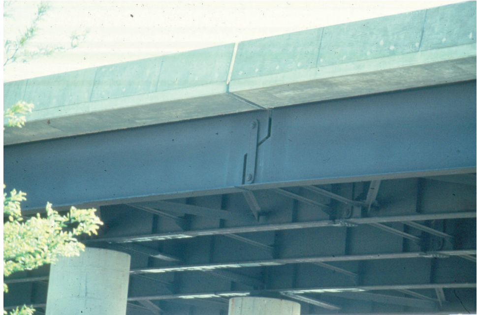
Figure 8.2.9 Fabricated Multi-girder Bridge with Pin & Hanger Connection
