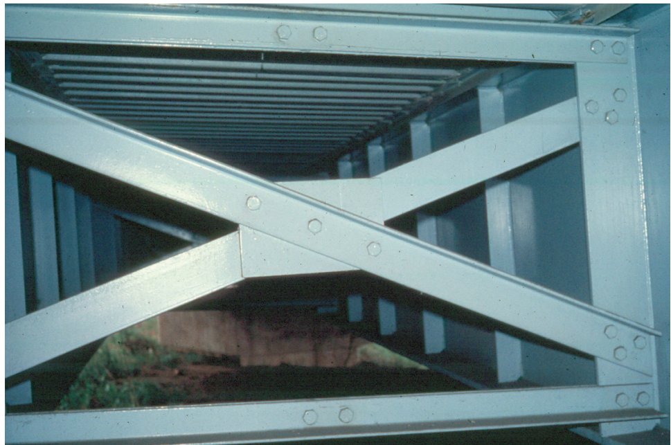
Figure 8.2.22 Intermediate Diaphragm
