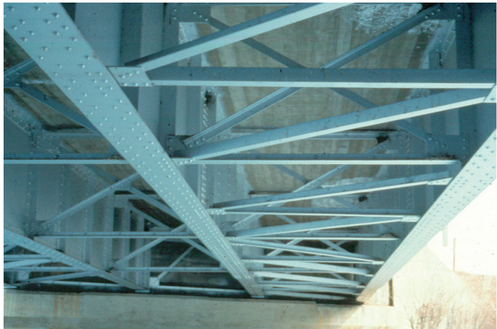
Figure 8.2.15 Straight Multi-girder Bridge
