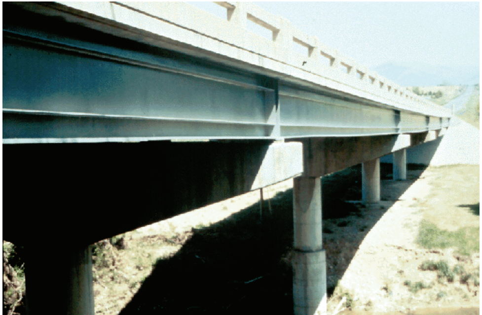
Figure 8.1.4 Structurally Redundant Continuous Span Bridge
