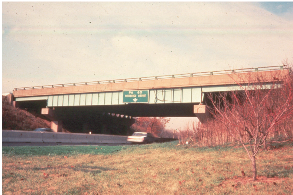
Figure 8.2.10 Combination Rolled Beams and Fabricated Girders
