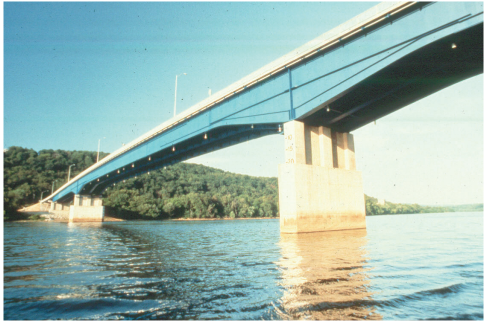
Figure 8.2.12 Fabricated Variable Depth Girder Bridge
