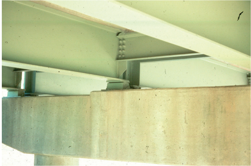
Figure 8.2.21 End Diaphragm
