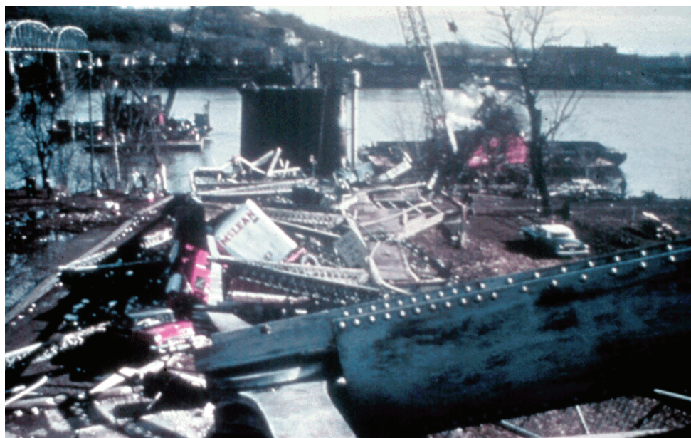
Figure 8.1.1 Silver Bridge Collapse
