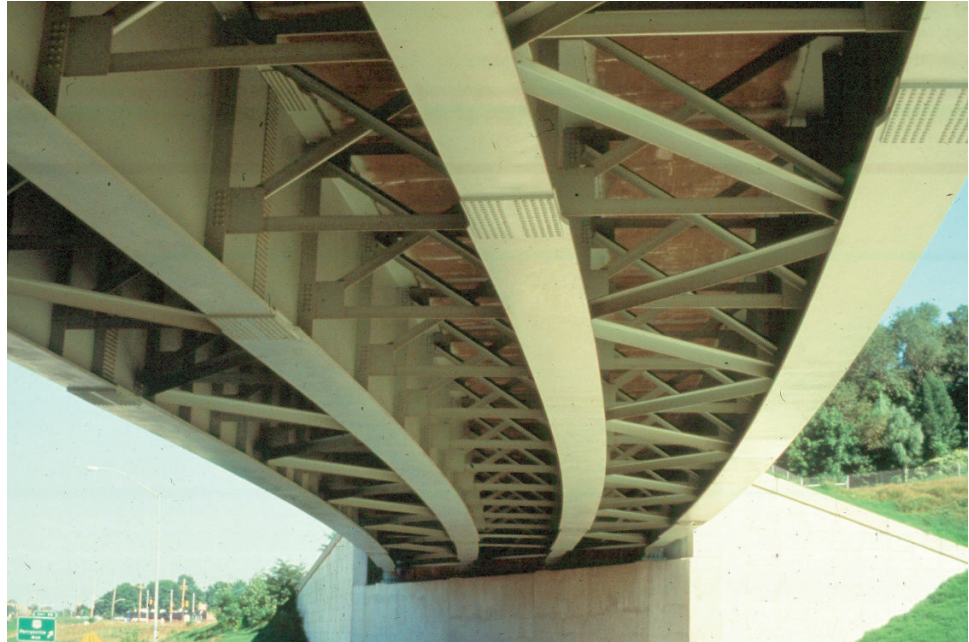
Figure 8.2.14 Curved Multi-girder Bridge
